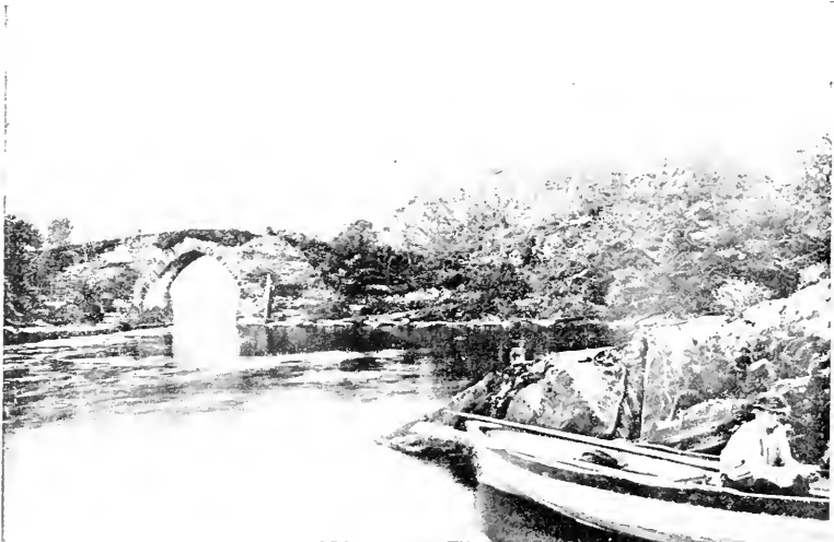
BRIDGE AT THE LAKES OF KILLARNEY, IRELAND.
